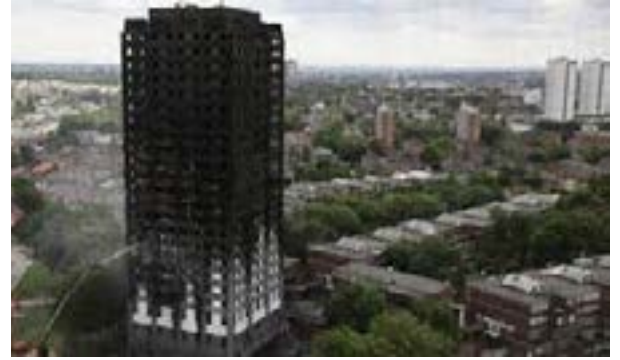
The burned-out hulk of Grenfell Tower looms over Kensington. (Photo: The Independent)
